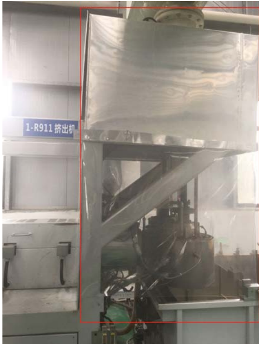
挤出废气集气罩
